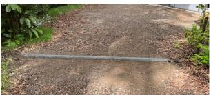
bought a steel pipe from the recycling centre for \$30 to divert the water into the bush. Roger started to dig a trench to take it but it was hard going in the compacted gravel. Geoff came along and said he had a jack hammer from his opal mining days. Ten minutes later the job was done! Thank you Geoff.
